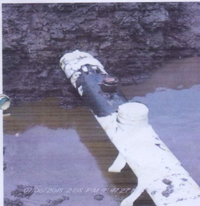
Fig C: Incident Facility after excavation
