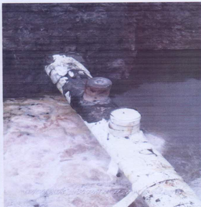
Fig D: Incident facility during repair
